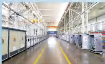
Electrical Complete Set Workshop
